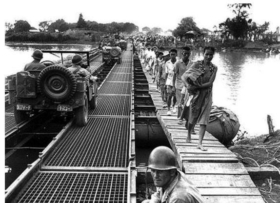
Photo of Nagtahan Bridge, February 1945.
