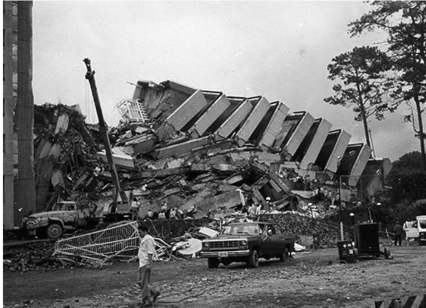
The Hyatt Terraces Hotel in Baguio was destroyed in the Luzon Earthquake of 1990. It was never rebuilt.
