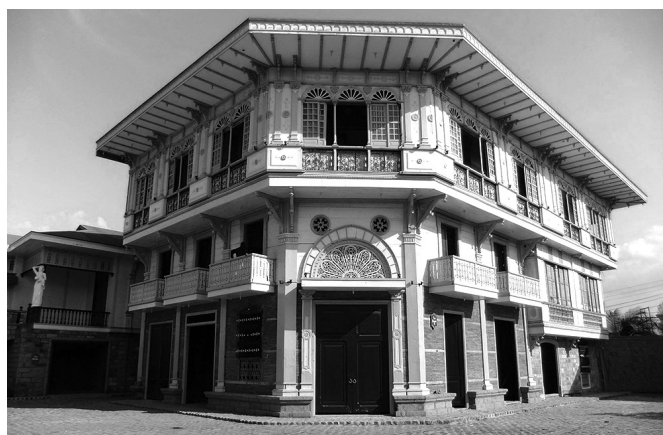
Casa Vyzantina, an ancestral house used to be situated in Manila, housed Instituto de Manila. The structure has been moved piece by piece and reassembled in Las Casas Filipinas de Acuzar, Bataan.
