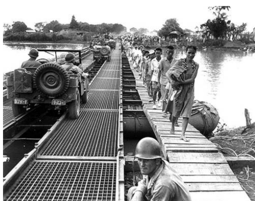
PHOTO: Nagtahan Bridge from Correos Filipinas Tumblr, February 1945. Photo courtesy of Manuel L. Quezon III.
